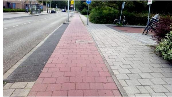
These entrance kerbs are arranged in a straight line as a continuation of the ordinary kerbs on the main carriageway, without any indentation which could suggest the beginning of a side road. In addition to specifying the use of entrance kerbs as a defining feature of an “exit”, Dutch guidance also specifies that there must not be any kerb corners which might imply the beginning of a section of carriageway.
