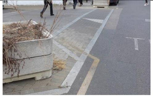
Note that other factors, beyond actual ramp design, also affect how easily a ramp is driven over. These factors include the degree of crossfall on the footway and on the carriageway, and any incline along the side road (as visible at Woodside Avenue and Scott Street in the images above).
