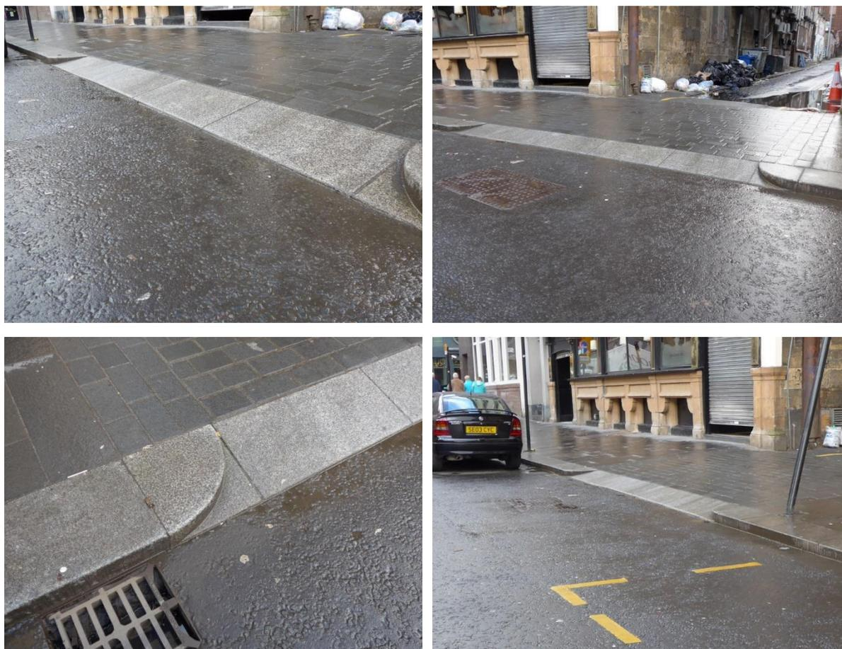
Local details mean that the height of the ramp varies a little at the other similarly constructed Glasgow designs. For example, at the junction of Anchor Lane with West George Street the kerbs sit higher compared to the surface of the carriageway, and higher at one end of the ramp than the other, meaning the ramp height varies from around 100-120mm in comparison to the carriageway.
